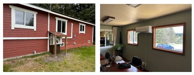
The do-it-yourself system installed at City Hall features one outdoor compressor unit and two indoor discharge units. The system heats both front and rear sections of the building comfortably even on very cold winter days.
